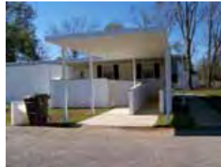
Uniontown Clinic Renovations
