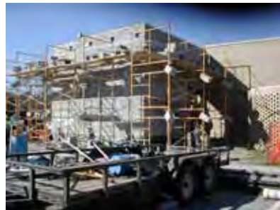
Construction of Houston County Health Department
