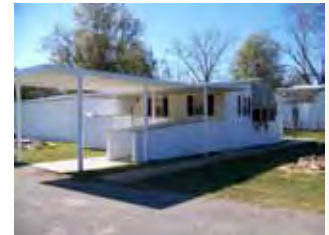
Uniontown Clinic Renovations
