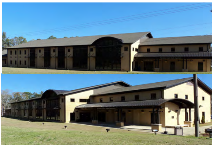
Two front views of the Main WIC site for Tuscaloosa County Health Department.
