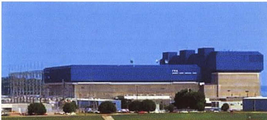
Browns Ferry Nuclear Plant on the Tennessee River, Limestone Co, AL
