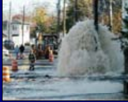
Staten Island Advance/Michael Oates Water is shooting out of the ground creating a lake on Richmond Terrace. 2008
